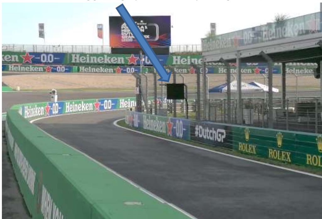
Figure 3 Pit Exit Road Light Panel
